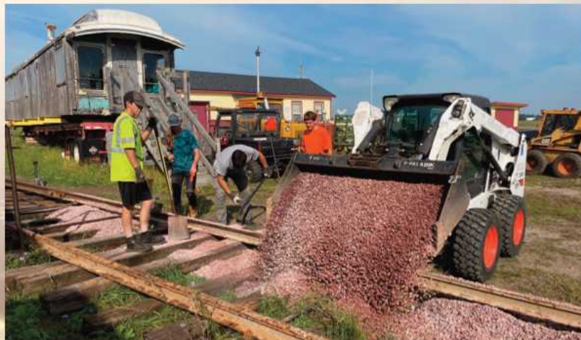
The Gopher State Railway Museum relies on a variety of volunteers to restore equipment and run its operations. At right, a load of ballast is poured into a section of railroad track.
